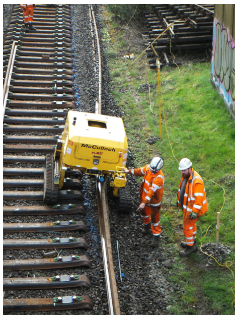
Railway works at Nymet Bridge, March 2026
